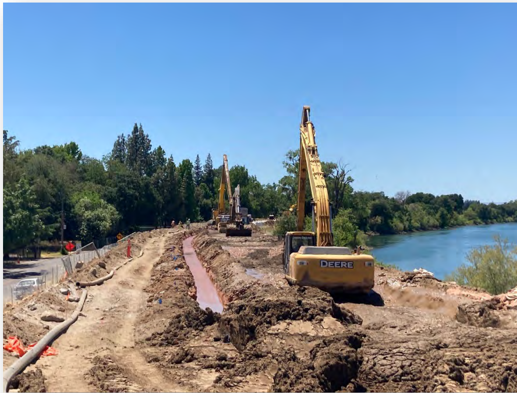
Soil/Bentonite Cutoff Wall
