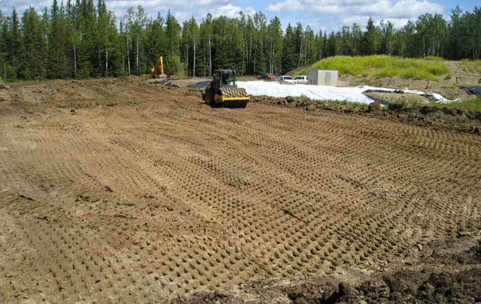
Compacted Clay Liner Construction
